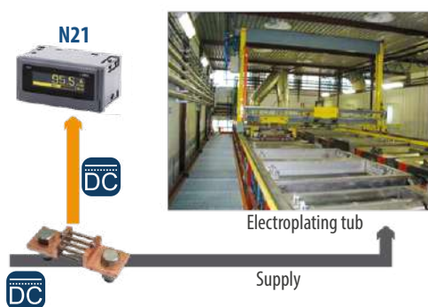
Current measurement in an electroplating plant
